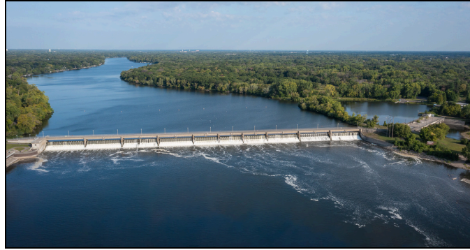
Figure 4.2.3: Coon Rapids Dam [46]
