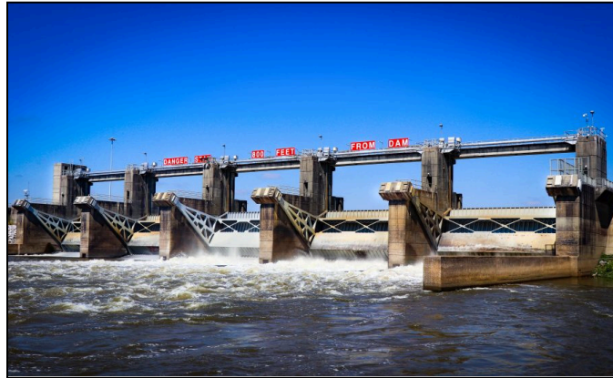
Figure 4.2.2: John C Stennis Lock & Dam [40]
